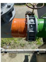
In many cases this can be a very long lasting repair, but as we often don't know the internal condition of the pipe it can also be seen as a temporary repair. In all cases it is a very strong repair that can withstand high pressures.
